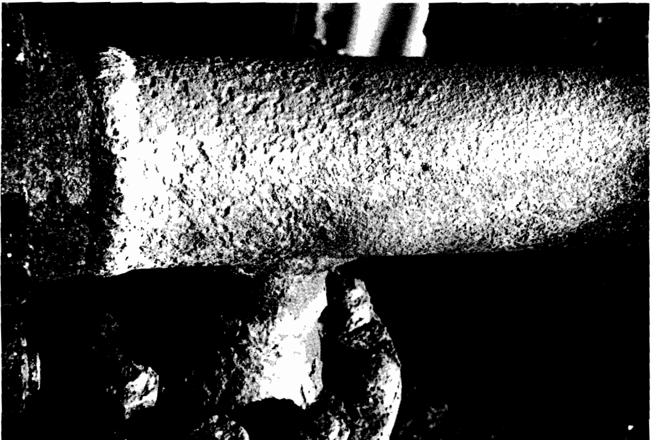
Figure 20—Severe Atmospheric Corrosion of Piping.
